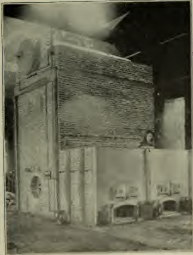
VIEWS OF THE CO. ORIGINAL WATER-TUBE BOILER IN THE STATE OF MICHIGAN
